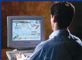
Line Control & Data Mgmt
